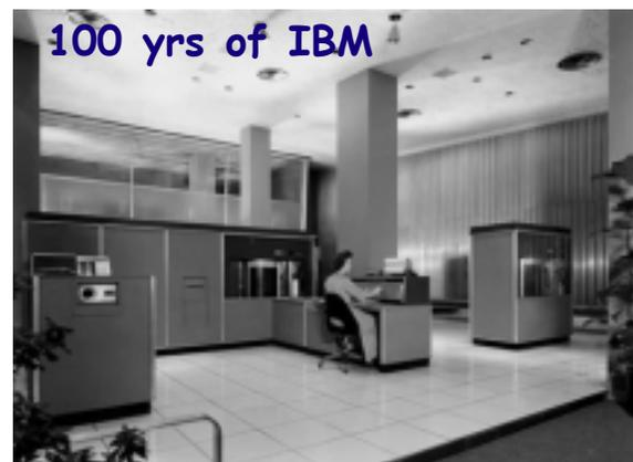
The Random Access Method of Accounting and Control (RAMAC) IBM RAM 305 from the 1950's, is shown. IBM was formed on June 16, 1911, as the Computing Tabulating Recording Co. in a merger of four separate companies. The new business with a plant in Endicott, N.Y., made scales, time clocks, cheese slicers and \_ significantly for its future \_ machines that read data stored on punch cards.
