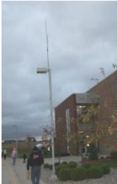
The antenna for the NECOS station was a plumber's delight J-pole elevated with a 25 ft pipe tied to a convenient light standard.
